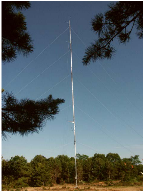
Figure 2 – 40 m data tower in Eastham during installation.
